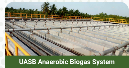
ETP - UASB Bio-Digester system
